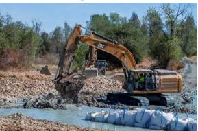
Workers plug a ditch dug by gravel-miners last century and redirect its water into a new channel on Clear Creek's original path. Credit: Brandon Honig/USFWS
