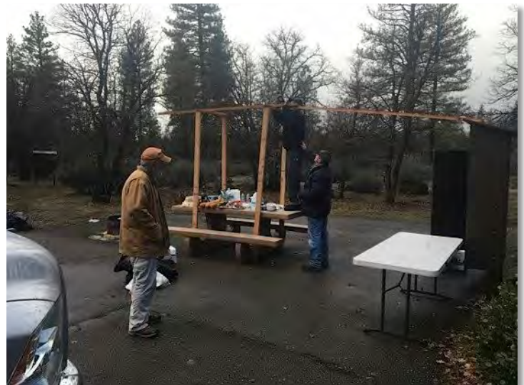
The secret was drilling into the asphalt
