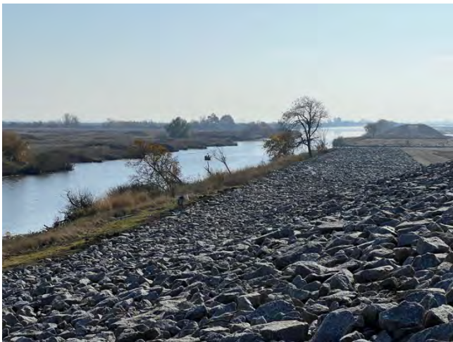
Riprap along the west side of Shag Slough looking south
