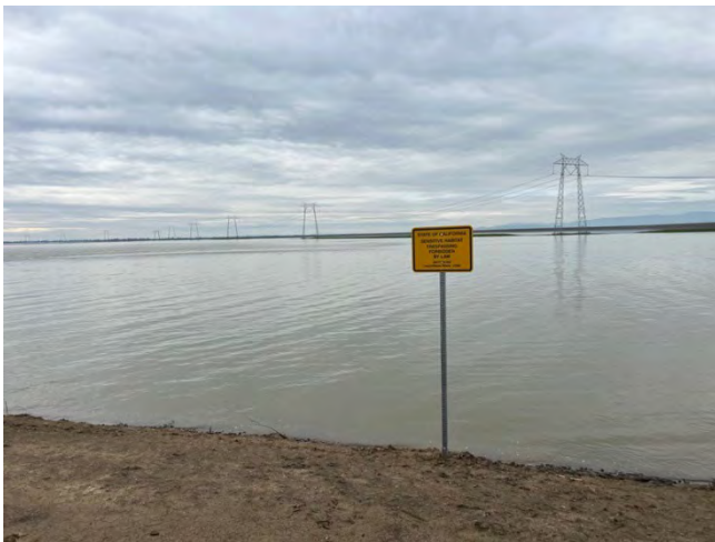
Looking west towards the new sloughs
