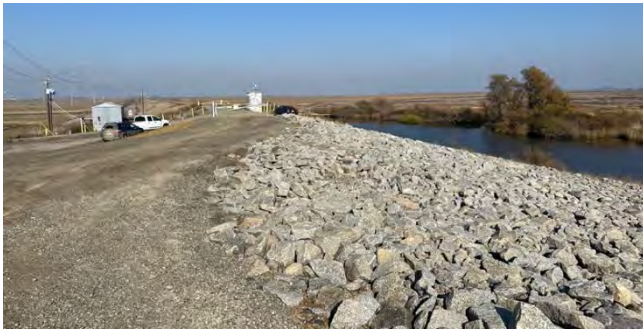
Looking north along Shag Slough
