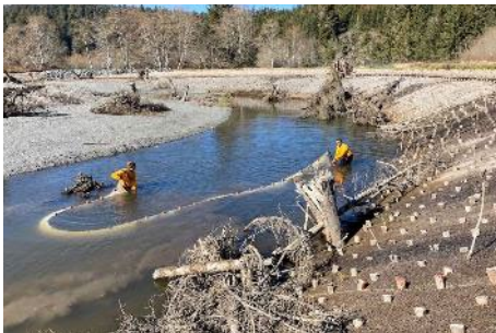
Prairie Creek Restoration Credit: Cal Poly Humboldt
